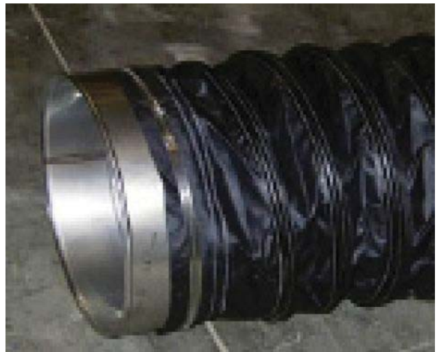
Duct (pn848172) installed on connecting band (pn848976) with 16" screw clamp (pn848176)
